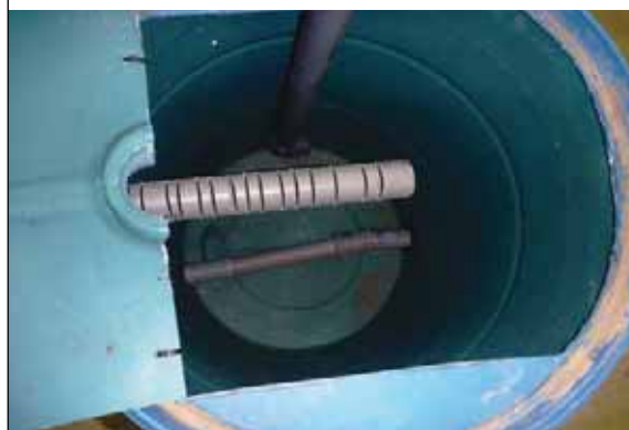
FIGURE 4.26 Picture of a mechanical solids separator
